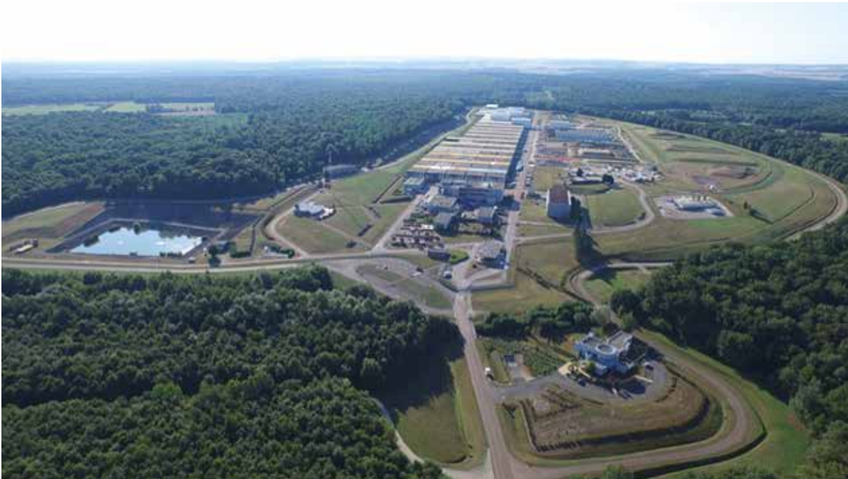
FIGURE 2 / AUBE STORAGE FACILITY (CSA)
