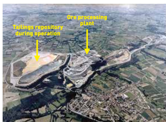
L'Écarpière site during operation (1989)
