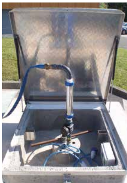
Piezometer used to take ground water samples
