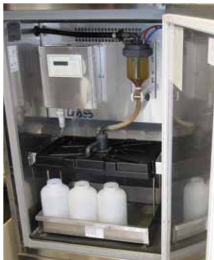
FIGURE 8 / WATER SAMPLING SYSTEM
