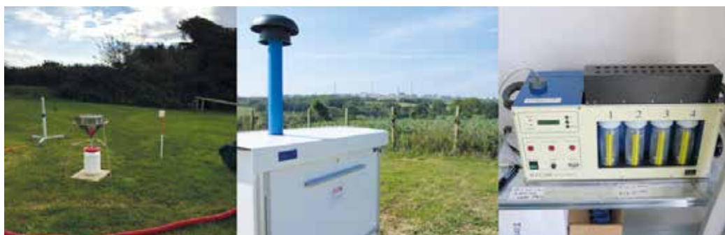
FIGURE A / INSTRUMENTATION INSTALLED AT THE IRSN SAMPLER AT OMONVILLE-LA-PETITE
